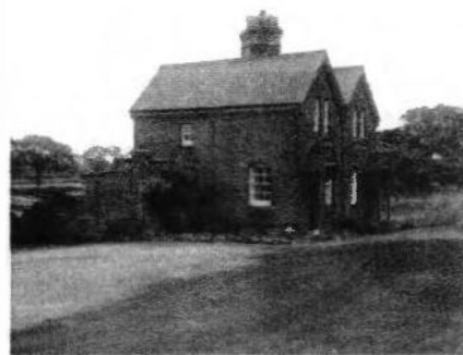
Another of Arthur Willis' photos of Mickle Trafford C.L.C. station, showing the two railway cottages in the goods yard in April 1968. They lasted until demolition in 1970.
