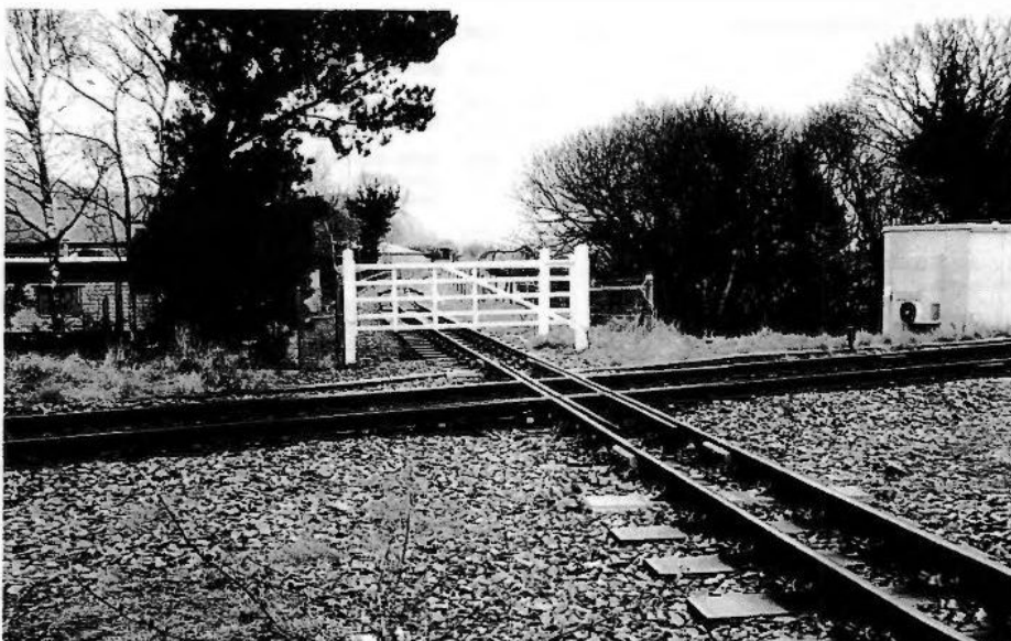
Where the standard-gauge Cambrian Coast line and the new 2ft gauge Welsh Highland line cross, on the level, on the outskirts of Porthmadog. Photographed by Tony Robinson on 2 March 2009.
