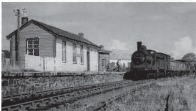
Whauphill Station – a timber structure which might well have matched the appearance of the original Whithorn Station prior to the construction of the later stone building Picture taken from Branches and Byways SW Scotland – Oxford Publishing Co
